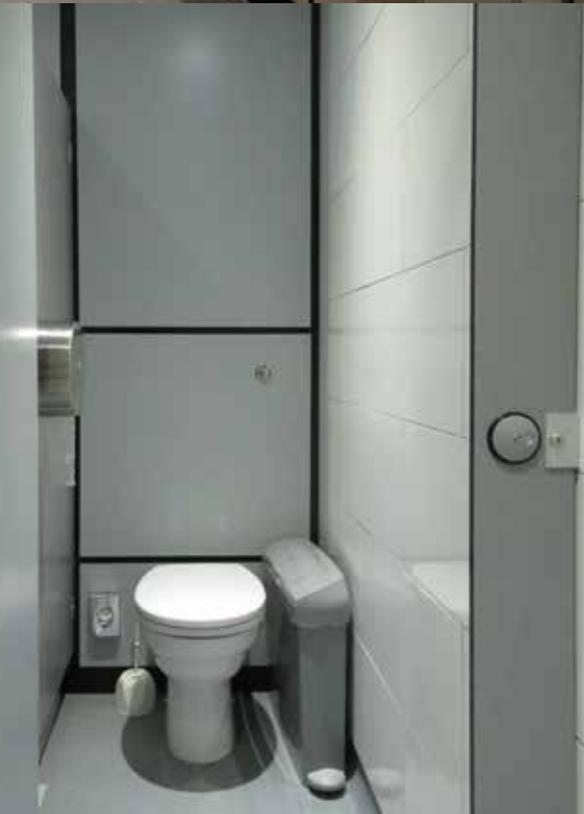
IPS duct panels (Integrated Plumbing System) allow for quick on-site installation coupled with clean-cut lines and a modern look.
